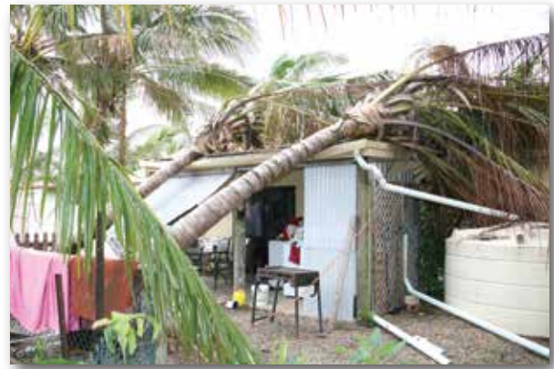
These palms landed on the roof during a storm due to severe root ball undercut caused by prolonged excessive use of Round-Up
